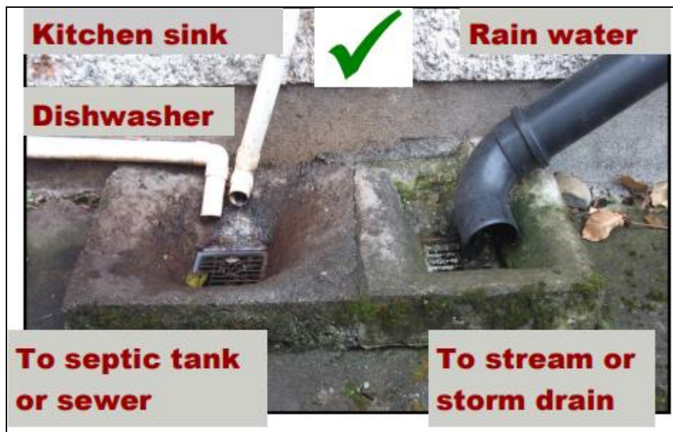
Figure 30. Correctly plumbed premises.
