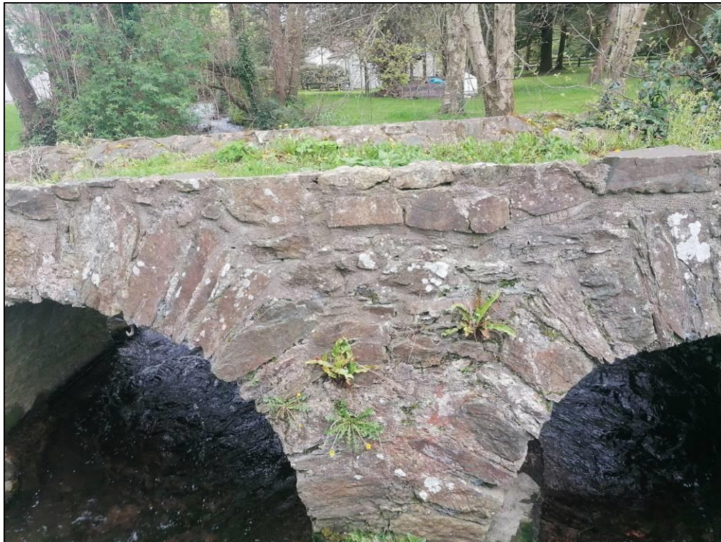
Plate 1. Possible Medieval Bridge over the Newcastle River on Temple Lane.
