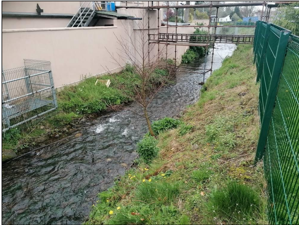
Plate 15. Development on the bank of the river. Note general lack of cover and riparian vegetation.
