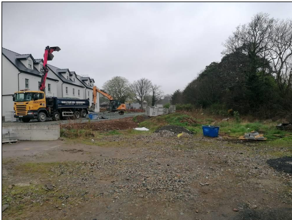
Plate 16. Construction works at Chancel Way.
