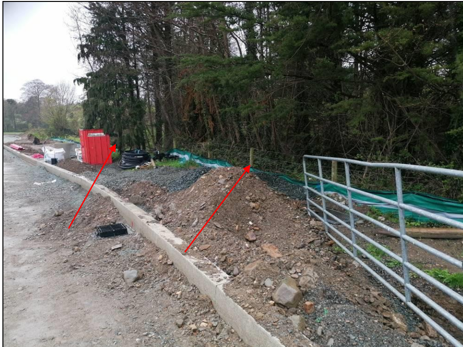
Plate 14. Silt fence adjoining the construction access road in Oaklawn.
